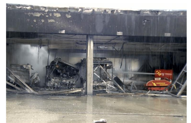
EV Bus Fire Damages Depot
