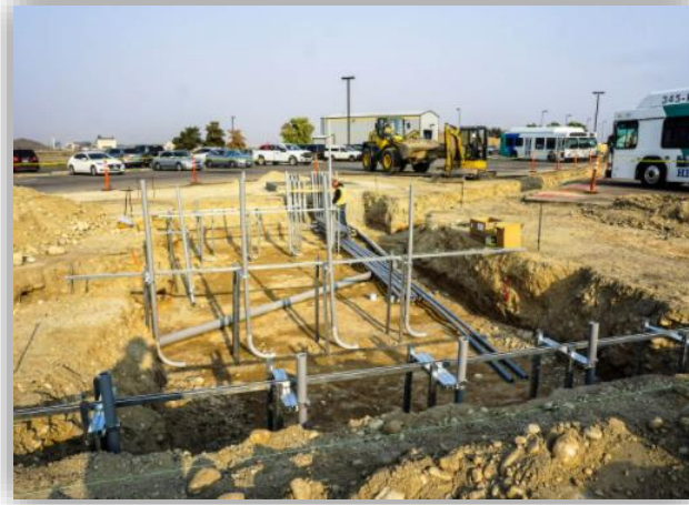
Reduced Parking - During Construction
